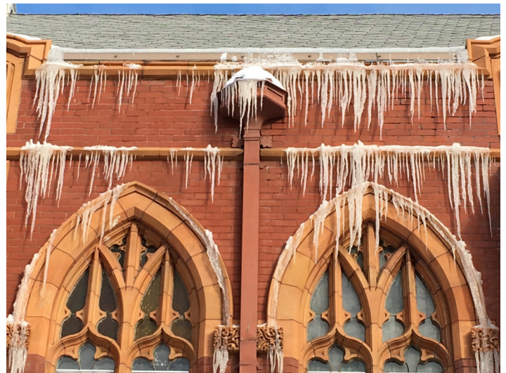
Before the restoration work began.
