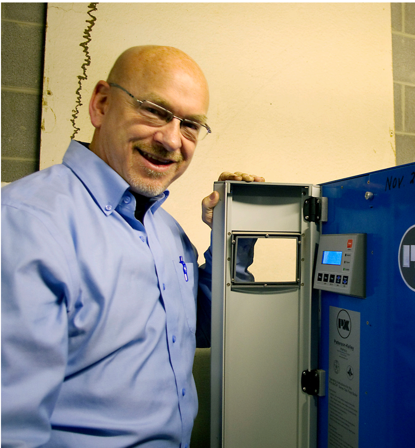
Terry Williams, STF Building & Maintenance Supervisor with new high efficiency boiler
