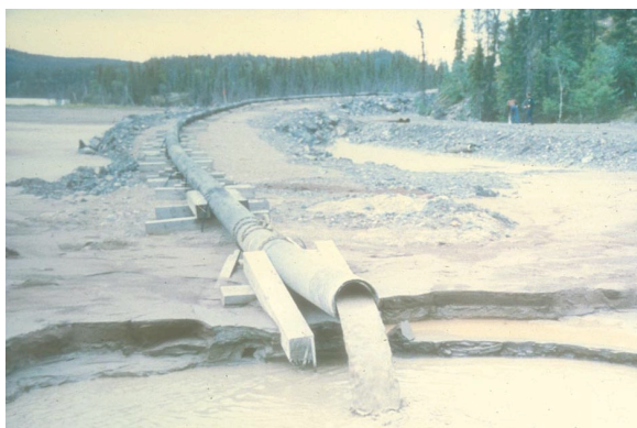
Outlet pipe from the Beaverlodge uranium mill near Uranium City, where vast quantities of radioactive waste were dumped into Fookes Lake, converting it into a tailings reservoir. The tailings reservoir lies in the Fulton Creek watershed (early 1980s).
